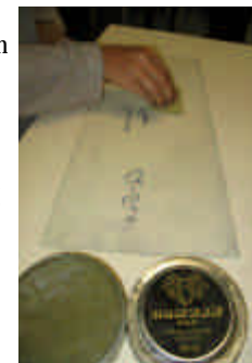
Mix about 10ml of resin. I use LR20 resin with LH137 hardener, which cures fairly quickly, giving about 10 minutes of pot life and a few hours to cure. My preferred method is to use a syringe to get the correct proportions as a scale is not accurate enough.
